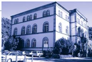
Altbau Tharandt (Main Building)
