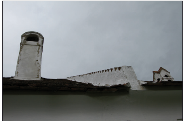
Chimneys with openings across the wind are elements of regional architecture in the Neusiedler See-Seewinkel area
