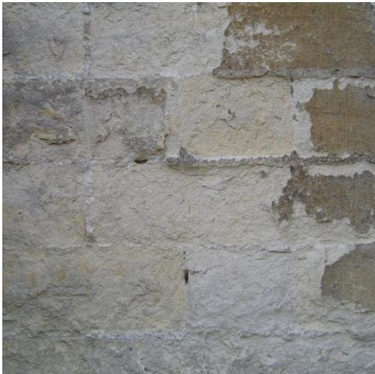
Degraded limestone due to acid rain
