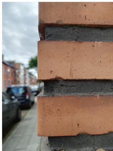
In case of recessed joints, the upper part of the bricks are less protected against rainwater.
