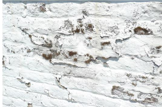
Degradation of a vapour-tight paint
