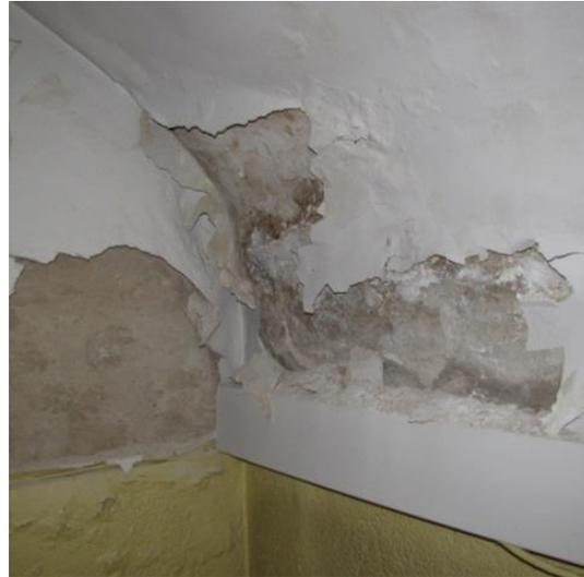
Coating and plaster are spalling off
