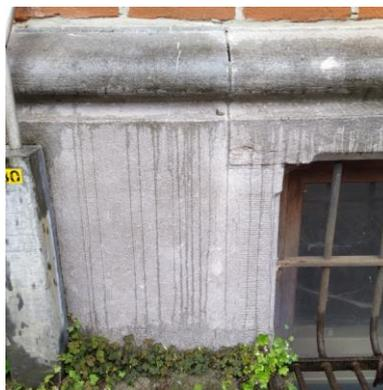
Visual indication of the presence of a water repellent agent: the surface cannot be wetted, water that runs off the façade forms fine runoffs or droplets.
