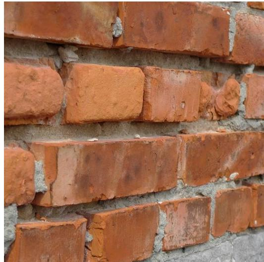
Damaged mortar joints
