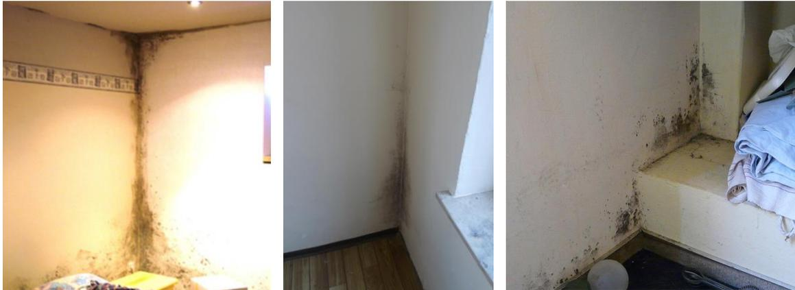
Fig. 13 Mould/condensation in the area of thermal bridges
