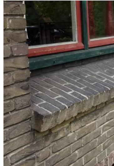
Brick window sills protect underlying wall less efficiently
