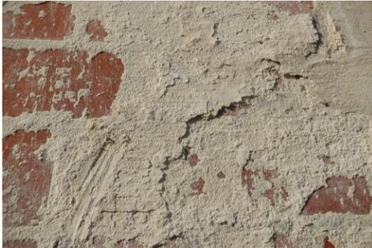
Degradation of a mineral paint
