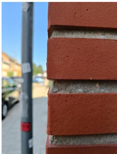
So-called 'shadow-joints' or 'Dudok-joints' offer less protection for infiltration of rainwater, as it has more time to penetrate the brick.
