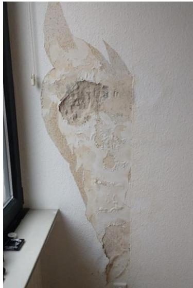
After removing wall paper visible mould stains
