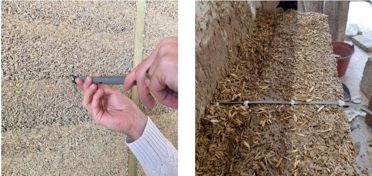
Figure 60: Installation of measuring probe in the wall, either using a PVC tube (left), or during construction (right)
