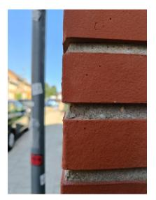
So-called 'shadow-joints' or 'Dudok-joints' offer less protection for infiltration of rainwater, as it has more time to penetrate the brick.
