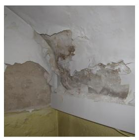
Coating and plaster are spalling off
