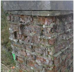
Cap stone does not stick, providing poor protection. Rainwater on the cap stone is absorbed by the masonry, which degrades.
