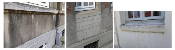
Fig. 7 Differences in pollution under a window sill. Left: apart from some runoffs, the surface under the window sill is well protected from water, as it is sooty; middle: cleaner surface under the sill, indicating it is exposed to rain; right: the runoffs of water under the sill can easily be observed
