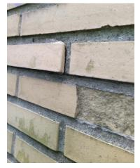
Glazed bricks (~1960s) degrading due to frost and limited drying potential of the masonry
