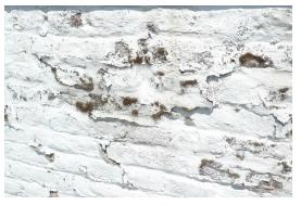
Degradation of a vapour-tight paint
