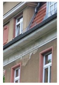
Discoloration on a facade under a rain gutter
