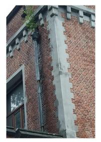
Water running over the façade due to a blockage
