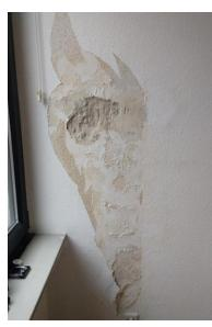
After removing wall paper visible mould stains
