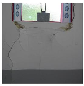
Degradation of plaster due to infiltrations through the façade
