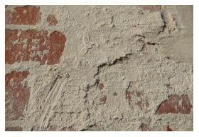
Degradation of a mineral paint
