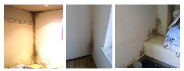
Fig. 13 Mould/condensation in the area of thermal bridges
