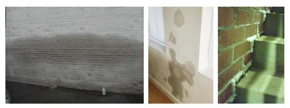
Fig. 12 Hygroscopic moisture and salts on an outer (left) and inner wall (centre); right: on the surface, salt crystallises out
