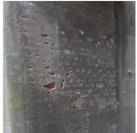
Damage to an exterior render, mainly due to salt crystallisation. The differences in porosity and pore size distribution between render, mortar and bricks give this specific damage pattern.
