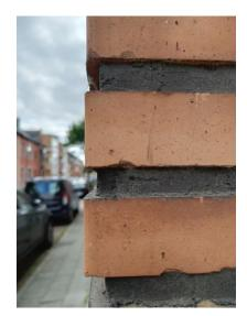
In case of recessed joints, the upper part of the bricks are less protected against rainwater.
