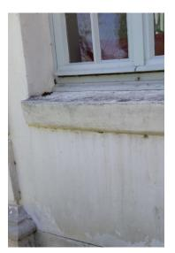
Water run-off on underlying wall demonstrate less efficient protection of non-ideal sill
