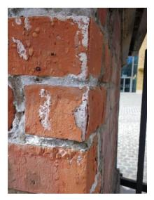
Loss of surface layer because of the application of a water repellent agent on a damp and salt-loaden wall
