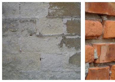
Degraded limestone due to acid rain
