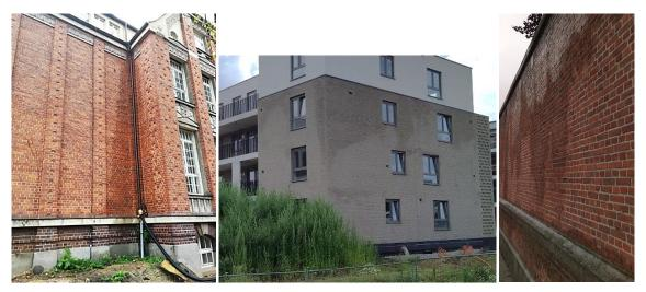
Fig. 5 Inspection after a rain event to visually check the moisture distribution on façade surfaces. Left: visible moisture load due to defective temporary rain water downpipe; middle/right: exposed parts become visible
