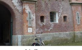
Salt efflorescence due to the drying out of a wall
