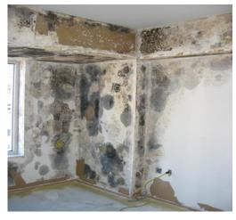
Fig. 14 Significant mould growth behind a removed PVC wallpaper (Wiss J. Elstner Associates, Inc.)
