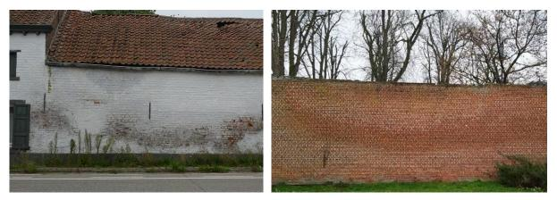
Fig. 11 Purely visually, it is not always easy to distinguish the moisture source. Left: dampening caused by rising damp. Right: dampening caused by hygroscopic salts
