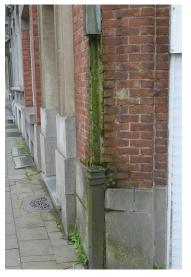
Algae and washed-out mortar due to missing rainwater pipe
