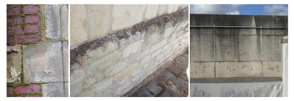
Fig. 6 Biological growth of moss, algae and bacteria showing where facades are exposed to rainwater
