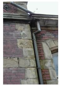
Algae and moss growth due to a defect external downpipe
