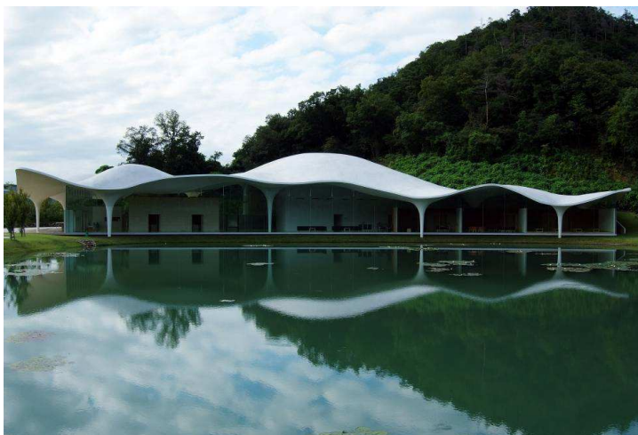
Bild. 1 Krematorium Kakamigahara, Toyo Ito and Associates [3] Fig. 1 Crematory Kakamigahara, Toyo Ito and Associates
