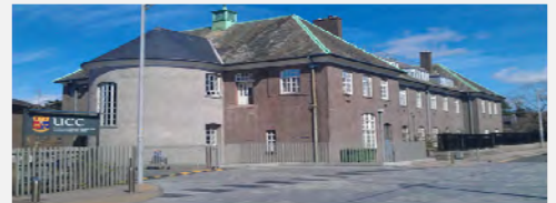
Figure 1. CEE building used as case study
