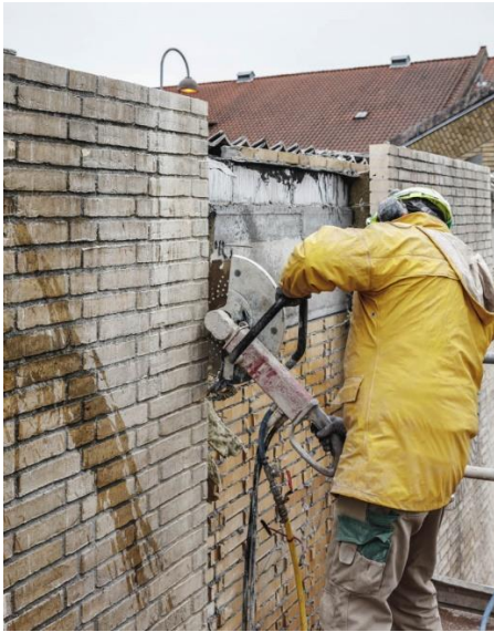
Figure 29: Cutting process of existing brick facades (Lendager)
