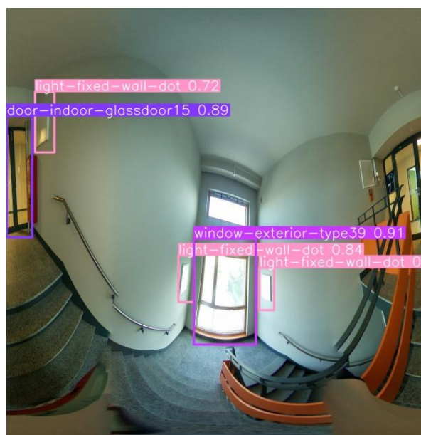
Figure 80 Sample image from batch 1 in the test set. The cut off part of 'door-indoor-glassdoor15' was not recognized in the right edge of the image. Furthermore, the smaller window above the 'window-exterior-type39' was not localized
