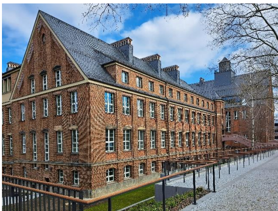
Figure 55: View of the Fritz-Foerster-Bau after ther renovation 2023.(Gebhardt, 2023), (CC BY-SA 4.0)
