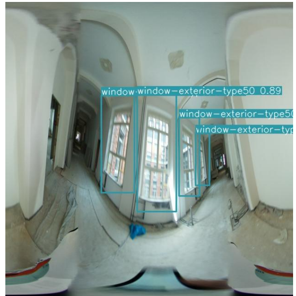
Figure 85 Image from batch 2 in test set. The labels of these windows are wrongly predicted as 'window-exterior-type50'. Since these windows have six cut-outs per sash in the central part, they correctly belong to the class 'window-exterior-type57'.
