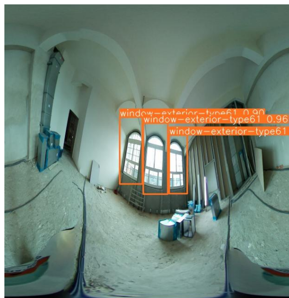
Figure 82 Sample image from batch 1 in the test set. The windows were correctly labeled as Type 61.83
