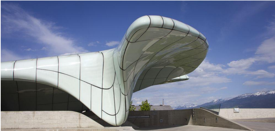
Figure 1.3 Double-curved glass panels with neoprene seal ( one of a series by Zaha Hadid, built for the Innsbruck in 2004) (Hadid 2007)
