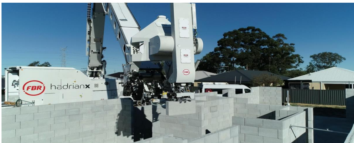
Fig. 7 – Hadrian X block-laying machine system source: https://www.fbr.com.au/view/hadrian-x
