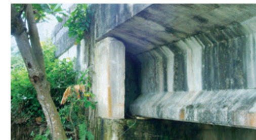
Longitudinal view of the bridge | Photo: AECOM – bridge inspection
