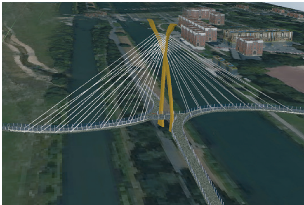
Conceptual design of the proposed cable-stayed bridge in Hamm | Graphic: Abdul Satar Aqaie
