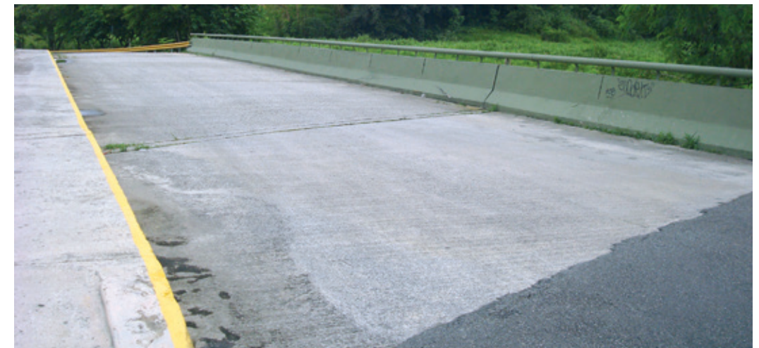
Top view of the bridge | Photo: AECOM – bridge inspection
