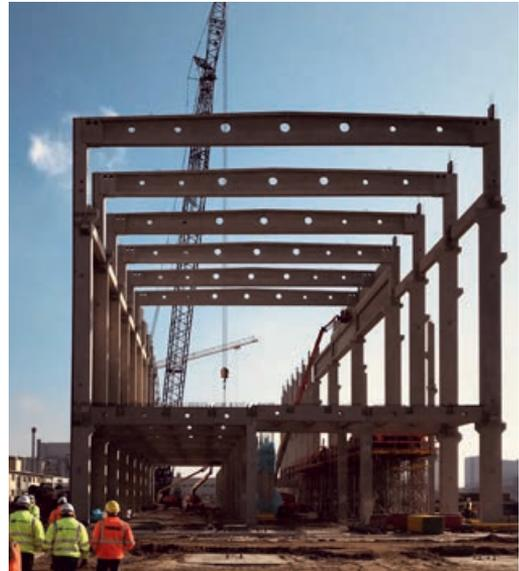
Precast elements with prestressing steel | Photo: Hentschke Bau GmbH, Bautzen
