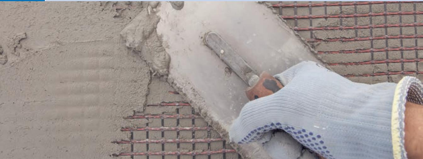
Einbau von Carbongelege | Installation of carbon reinforcement | Photo: Stefan Gräschel
