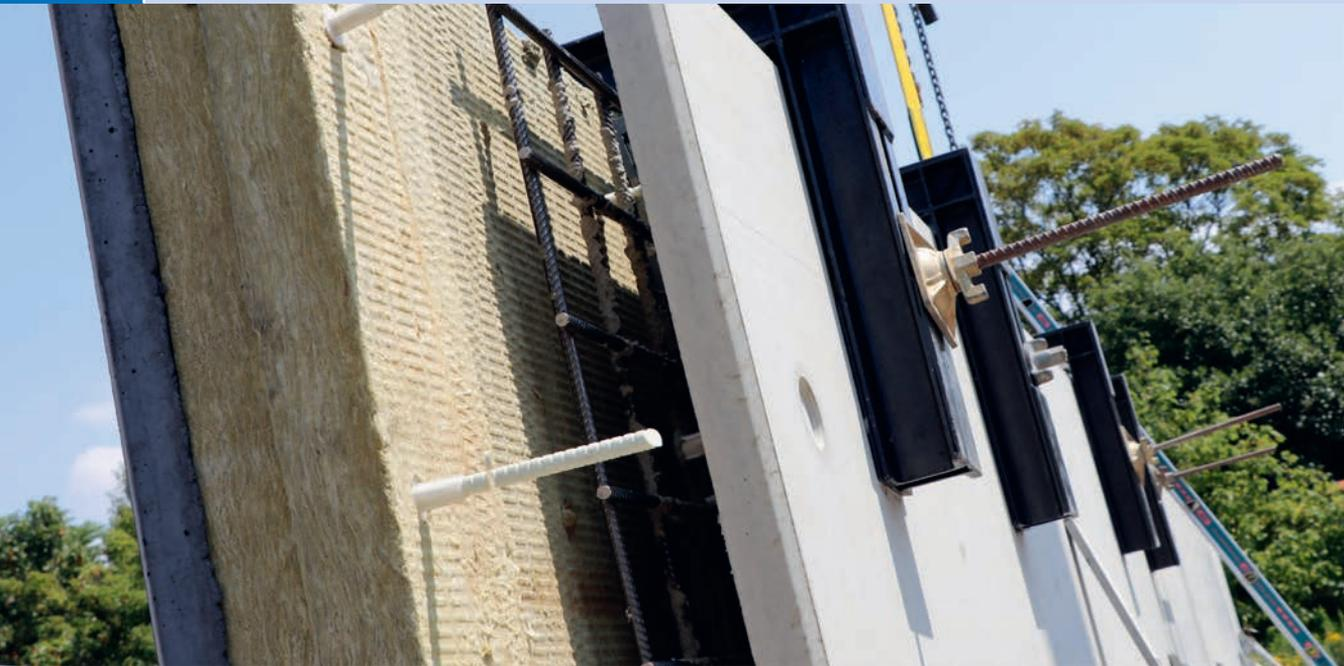
Elementwand aus Carbonbeton | Element wall made of carbon reinforced concrete | Photo: Matthias Tietze
