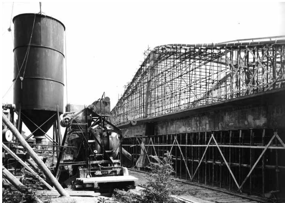
Fig. 8 Scaffolding of the bridge deck and the cables
