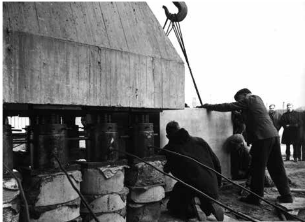
Fig. 6 Jacking up of the towers and positioning of the supporting concrete block
