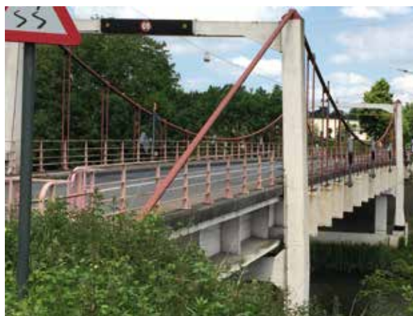
Fig. 9 First self-anchored suspension bridge (W13)
