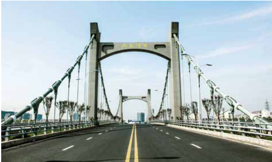
Fig. 13 Xiaolongwan Bridge in Nanjing (P.R. China)
