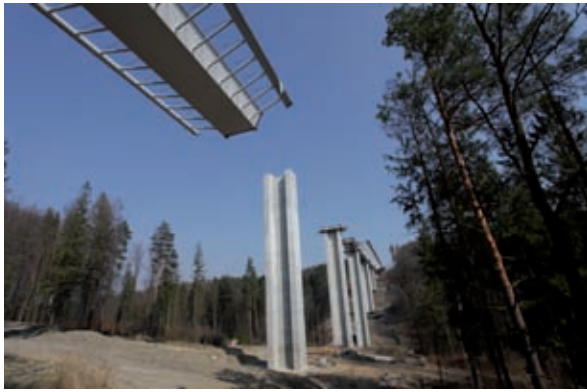
Fig. 15: Launching of the Bridge across the Kremlice Creek Valley (Photo: Jiri Dvorak)
