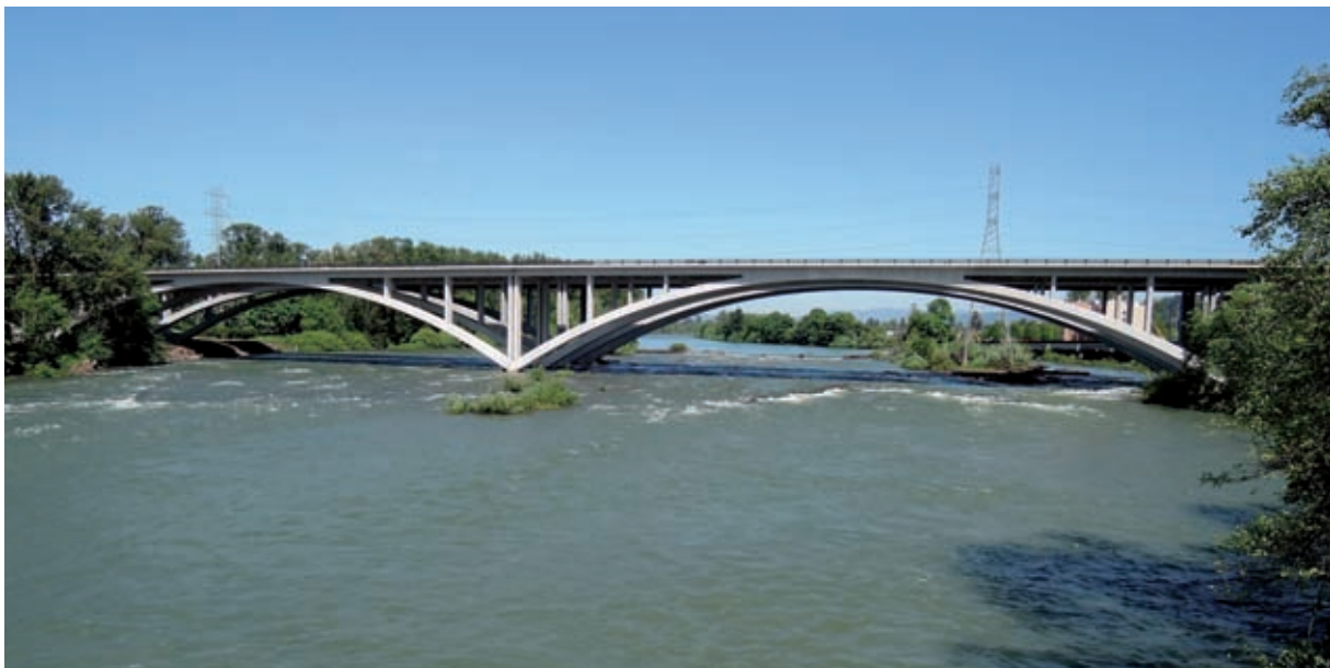
Fig. 22: Willamette River Bridge (Photo: Jiri Strasky)
