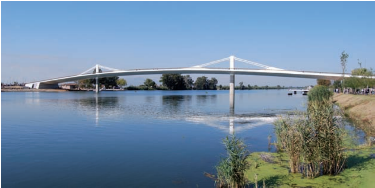
Fig. 24: Ebro River Bridge
