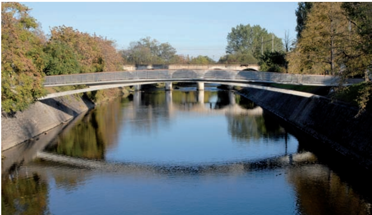
Fig. 30: Svatka River Bridge
