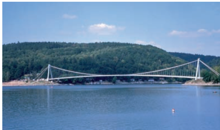
Fig. 3: Vranov Lake Pedestrian Bridge (Photo: Jiri Strasky)
