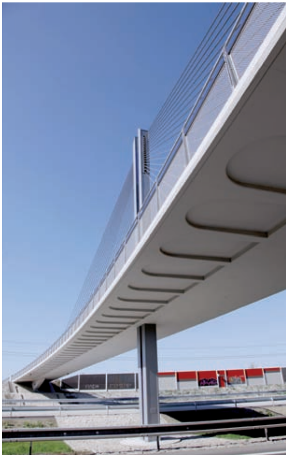
Fig. 25: Bohumin Drive Pedestrian Bridge
