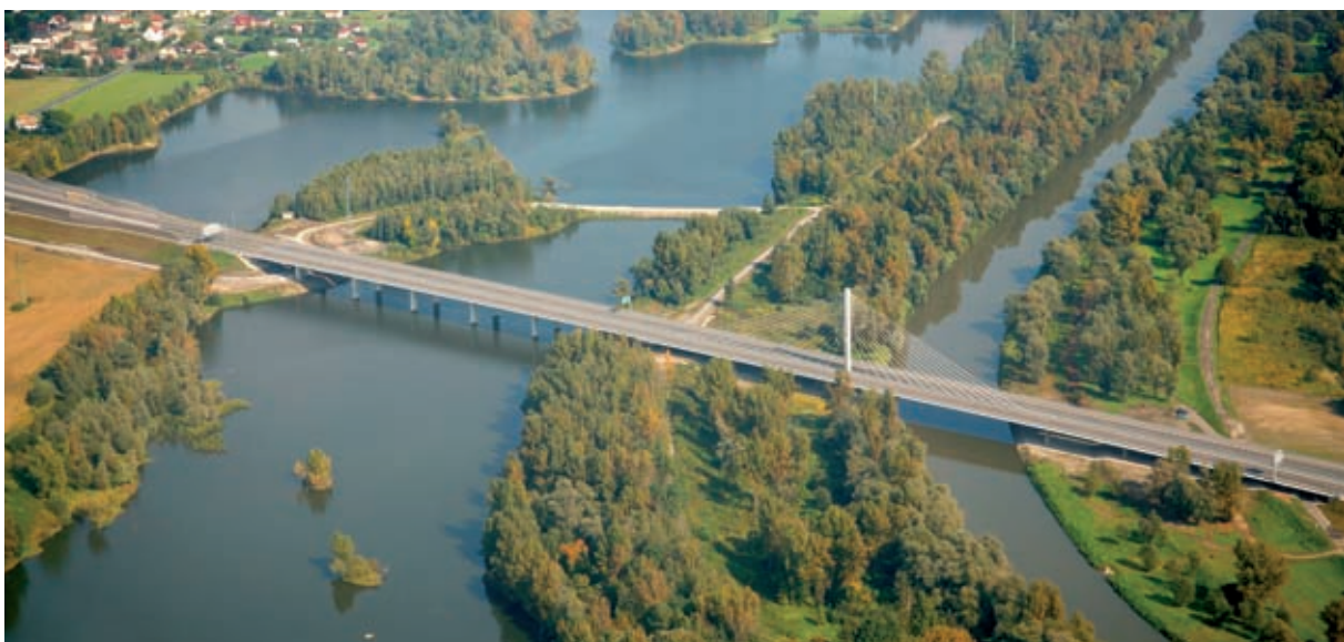
Fig. 23: Odra River Bridge
