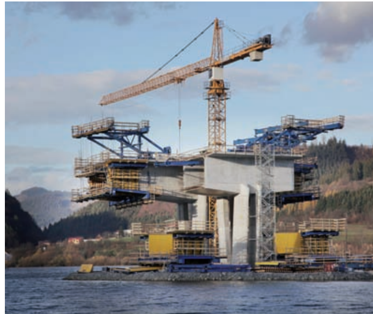
Fig. 18: Bridge across River Vah Reservoir Hricov (Photo: Jiri Dvorak)
