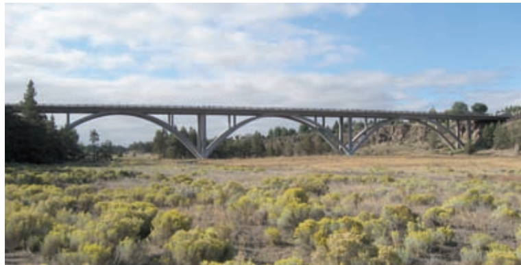
Fig. 21: Maple Avenue Bridge (Photo: Nadezda Straska)
