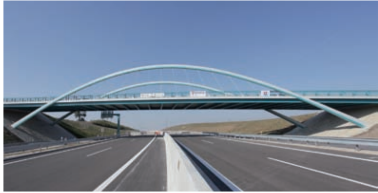
Fig. 20: Bridge across R1 near Nitra (Photo: Jiri Dvorak)
