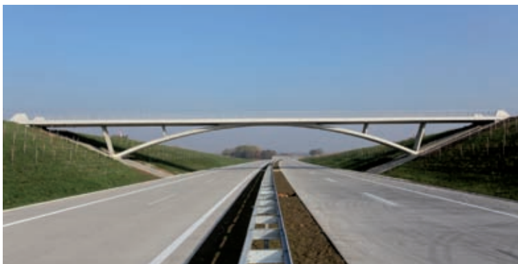
Fig. 19: Bridge across D1 near Studenka
