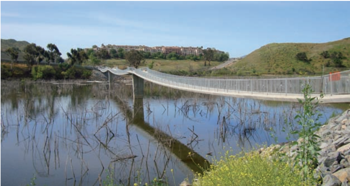
Fig. 28: Lake Hodges Pedestrian Bridge
