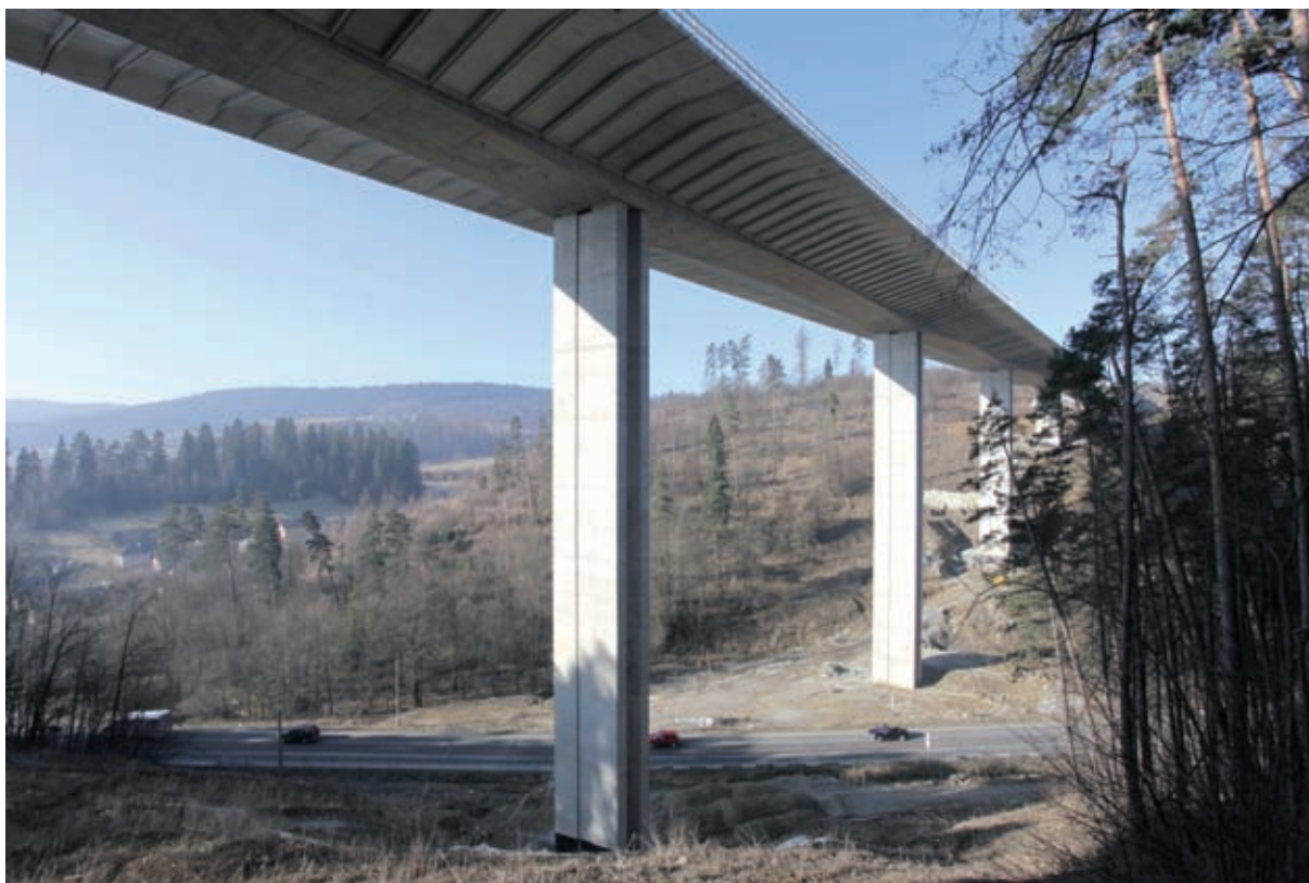
Fig. 12: Bridge across the Lodina Creek Valley
