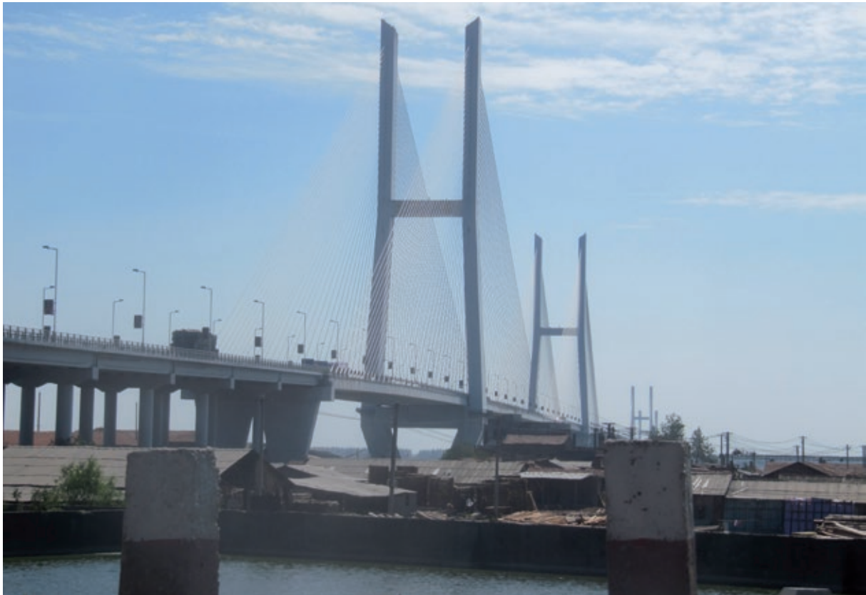
Fig. 7 Jingzhou Bridge across Yangtze River
