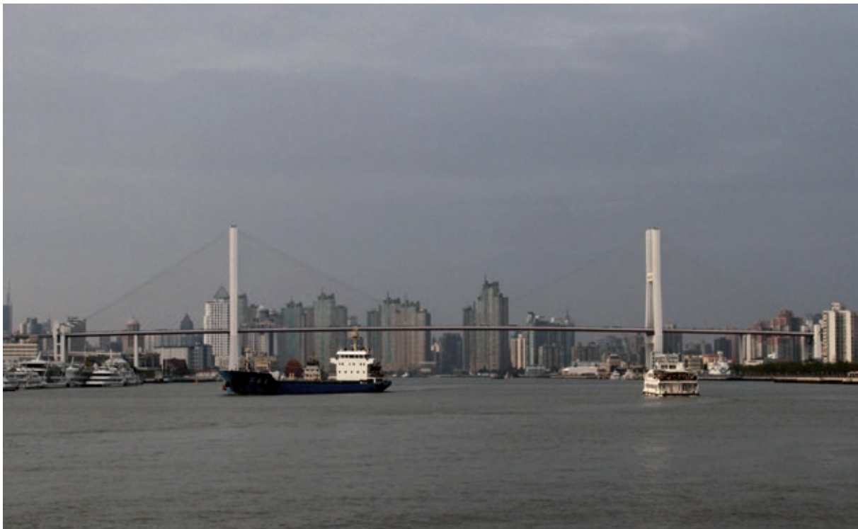
Fig. 1 Shanghai Nanpu Bridge
