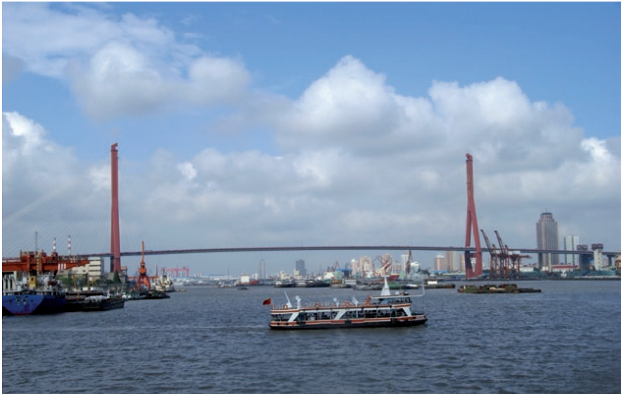
Fig. 2 Shanghai Yangpu Bridge
