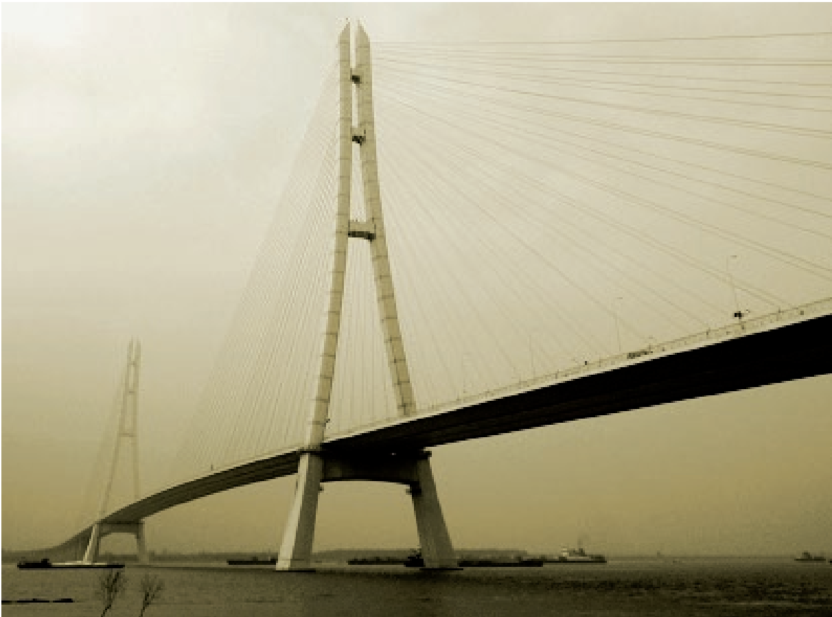
Fig. 4 Third Nanjing Bridge across Yangtze River
