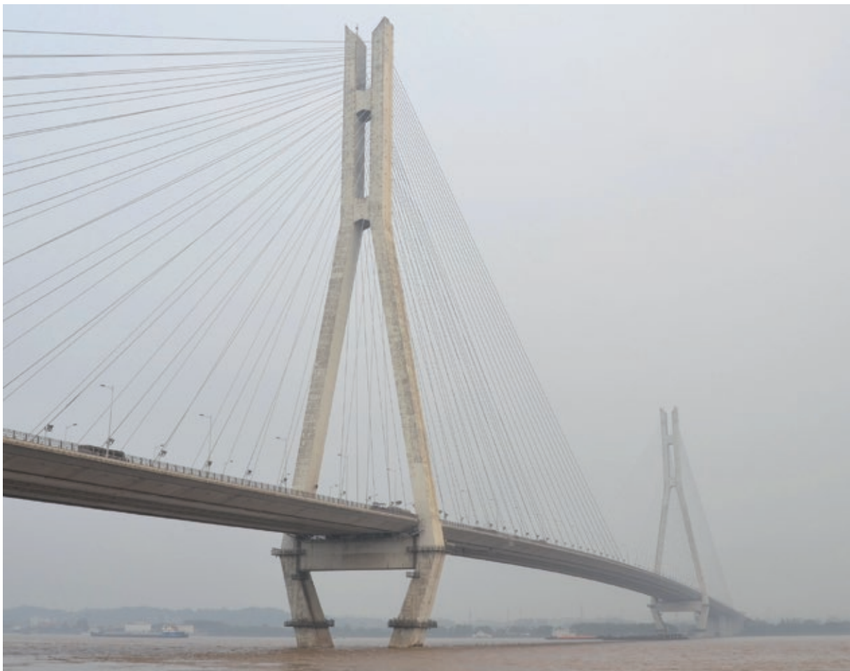
Fig. 3 Second Nanjing Bridge across Yangtze River
