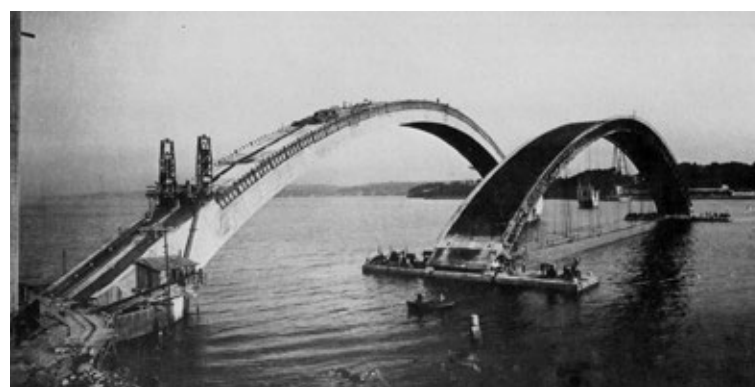
Figure 25 Centring of the Plougastel Bridge floating for the next arch
