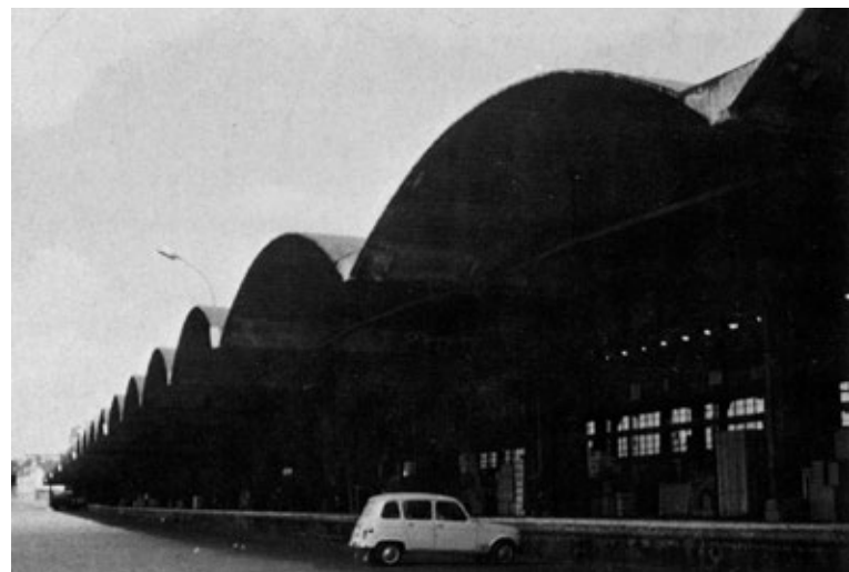
Figure 17 Vaults at the Gare d'Austerlitz, canopies
