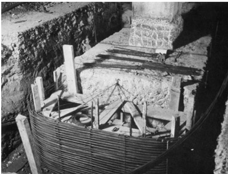
Figure 36 Anchor blocks at the Maritime Station of Le Havre, solution for rehabilitation by Freyssinet in 1934
