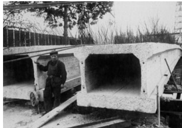
Figure 43 Luzancy Bridge, precast segments
