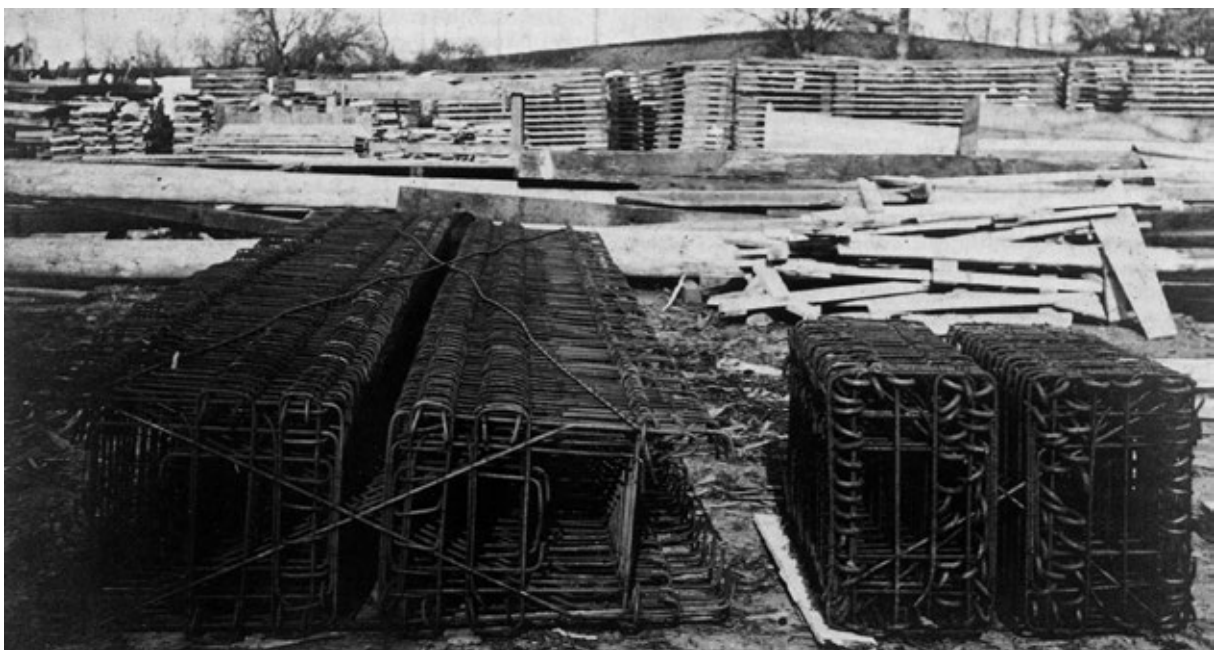
Figure 8 Boutiron Bridge, hinge reinforcement
