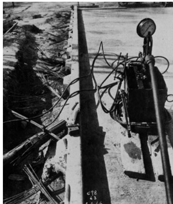
Figure 44 Luzancy Bridge, prestressing jack
