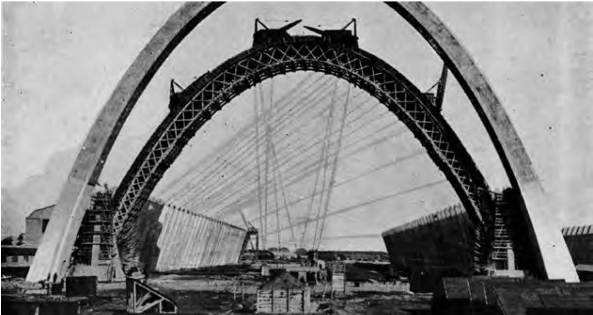
Figure 18 Orly Hangars during construction
