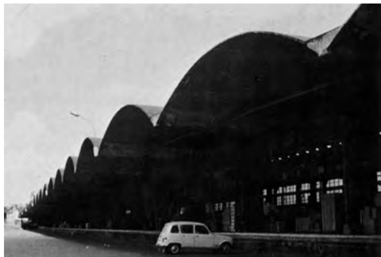
Figure 17 Vaults at the Gare d'Austerlitz, canopies
