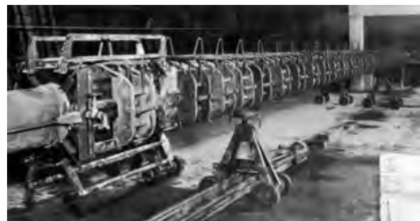
Figure 33 Flexible moulds to produce posts
