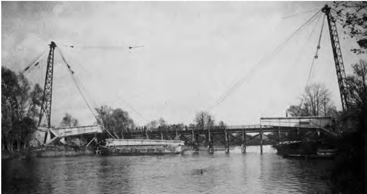
Figure 45 Luzancy Bridge, erection
