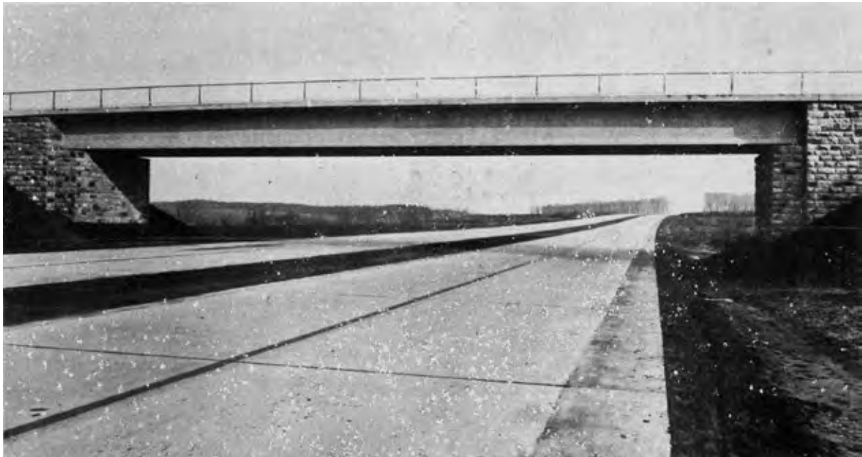
Figure 40 Oelde Bridge made with prestressed beams using Freyssinet's developments
