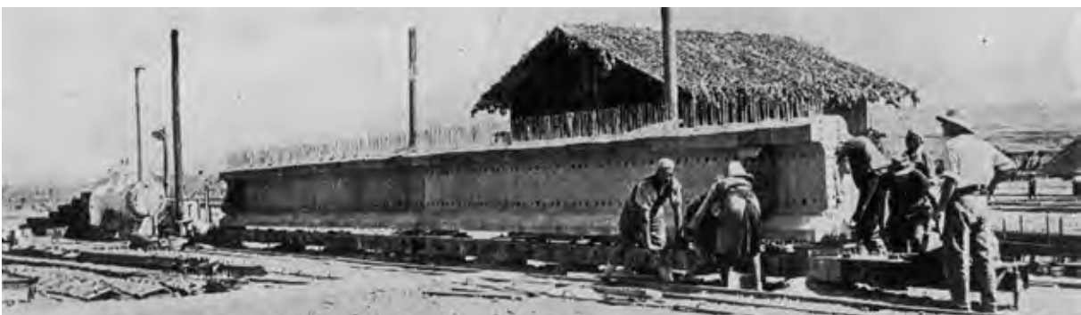
Figure 39 Precast prestressed beams for the Portes de Fer Bridge
