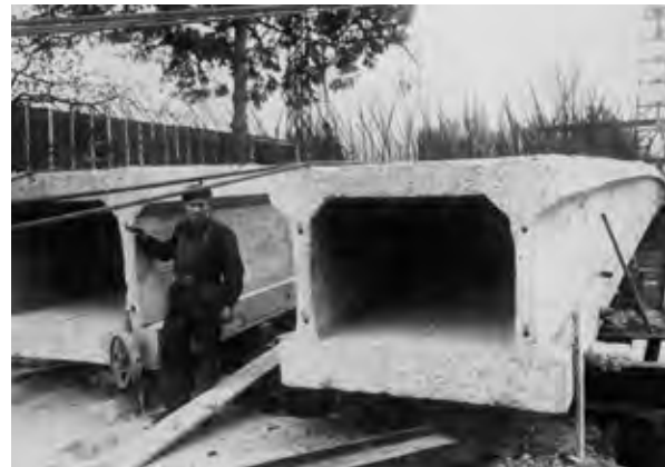
Figure 43 Luzancy Bridge, precast segments
