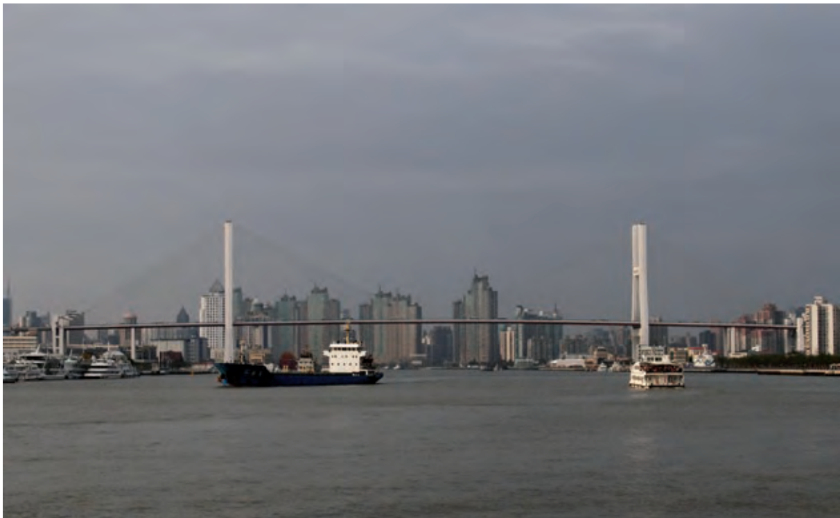
Fig. 1 Shanghai Nanpu Bridge
