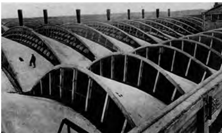
Figure 14 Conoidal vaults of 50 m span at the Factory for the National Radiator Company, 1928
