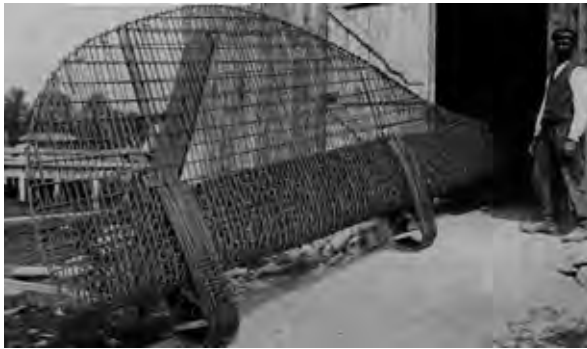
Figure 12 Reinforcement of a rudder for a reinforced concrete boat
