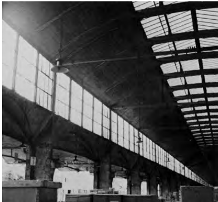
Figure 16 Vaults at the Gare d'Austerlitz, central vaults
