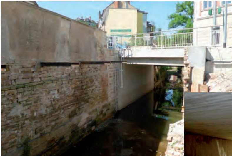
Mühlgrabenbrücke in Zeitz
