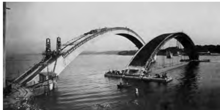
Figure 25 Centring of the Plougastel Bridge floating for the next arch
