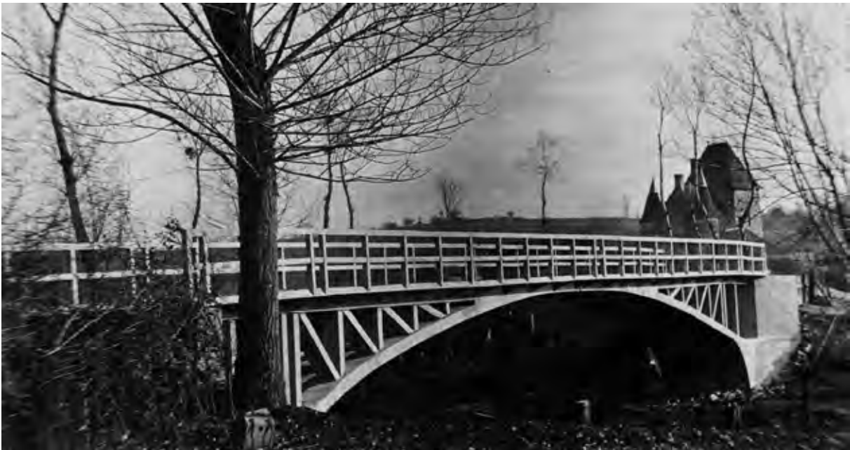
Figure 6 Bridge at Prairéal-sur-Bresbe
