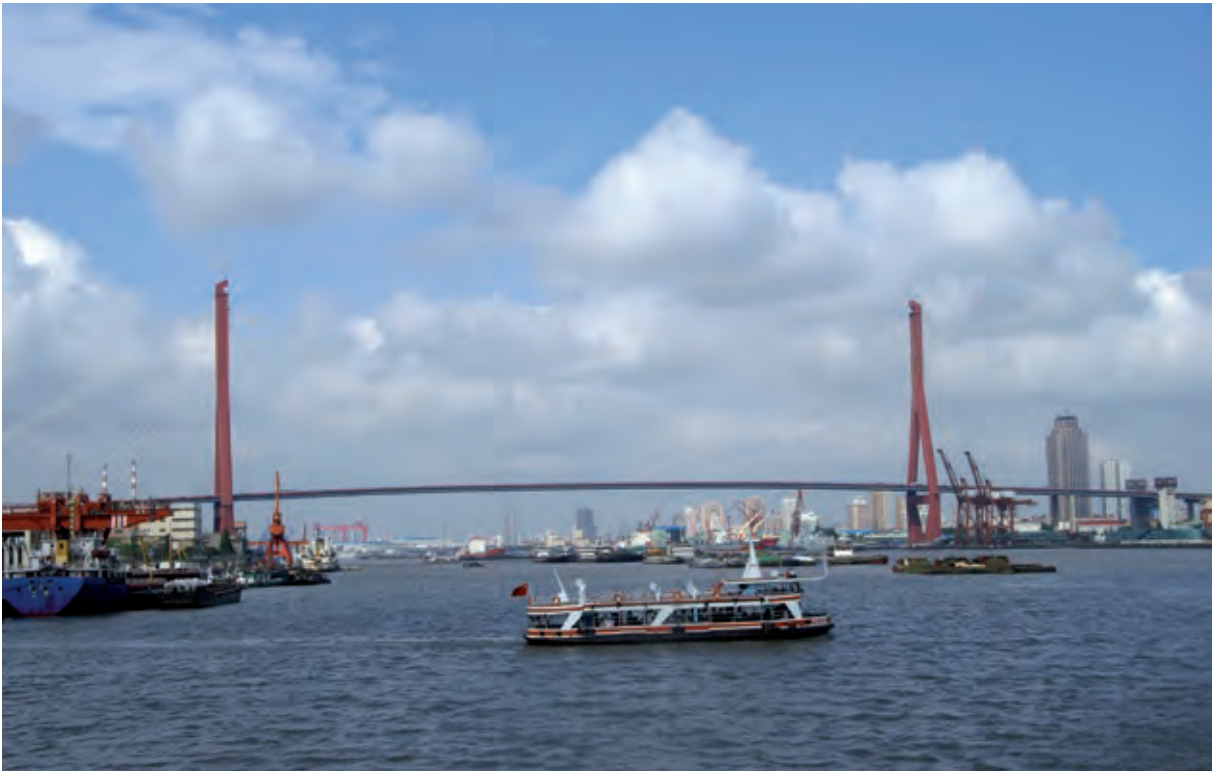
Fig. 2 Shanghai Yangpu Bridge
