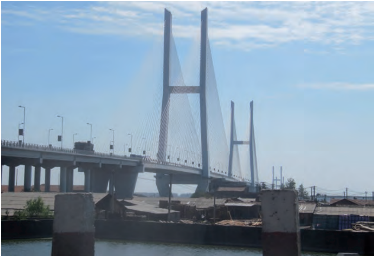
Fig. 7 Jingzhou Bridge across Yangtze River
