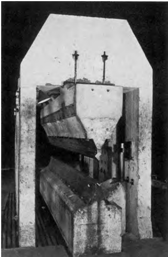
Figure 30 Prestressing press at Montarguis
