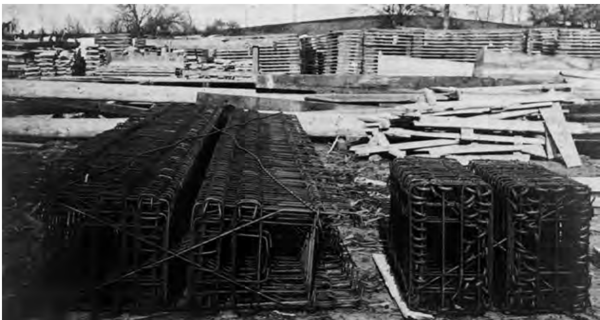
Figure 8 Boutiron Bridge, hinge reinforcement
