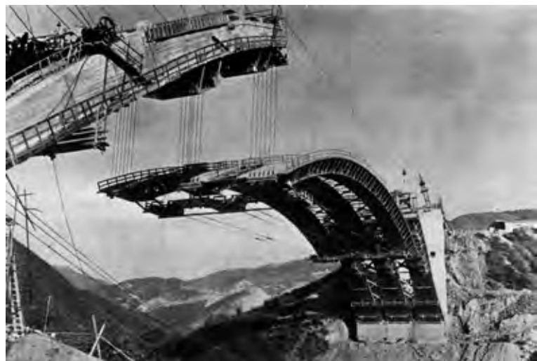
Figure 46 Viaduct at La Guaira Highway, centring
