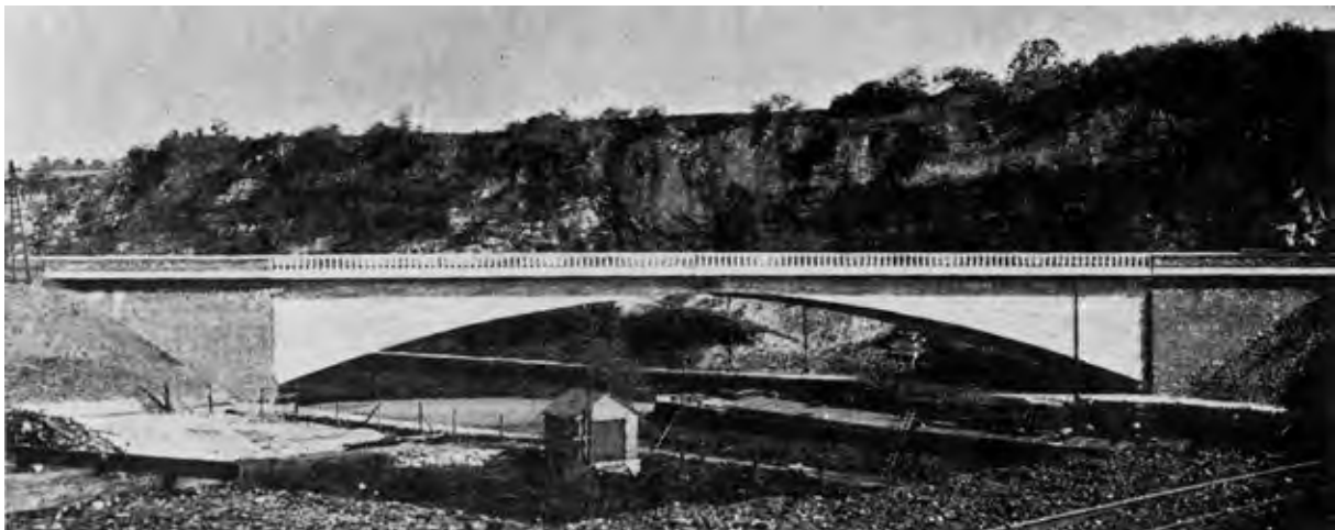
Figure 22 The Candelier Bridge
