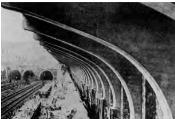
Figure 4 Cantilevers built by Rabut in Rue du Rome in Paris with stressed bars
