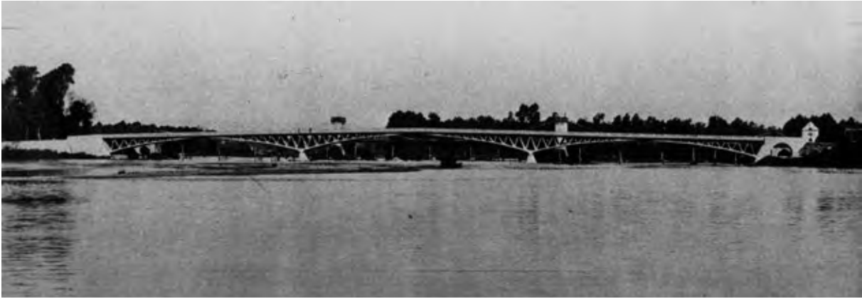
Figure 10 Le Veudre Bridge
