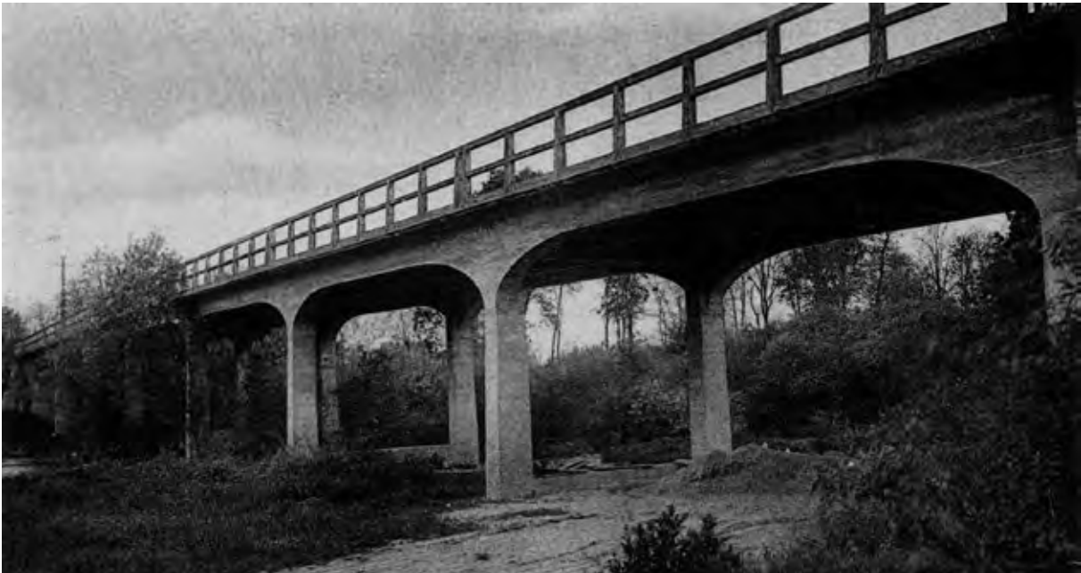
Figure 5 Bridge at Dampierre-sur-Besbre
