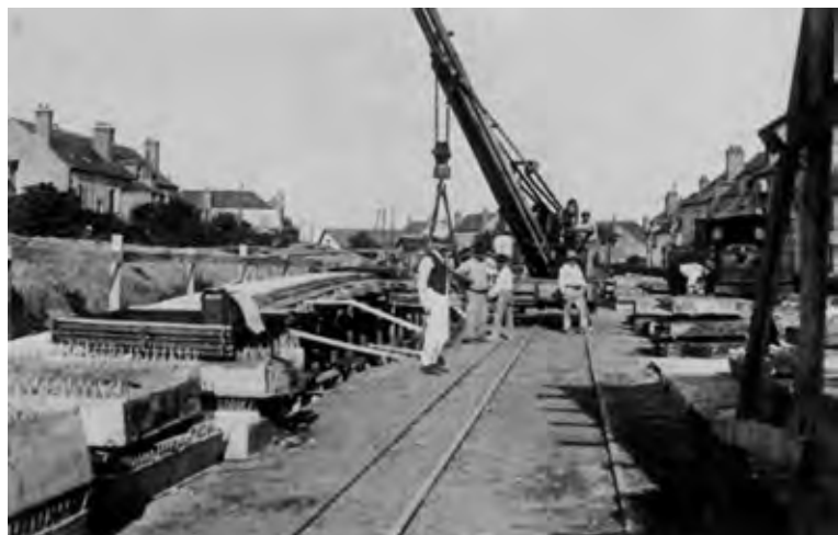
Figure 27 Test arch of the Veudre Bridge
