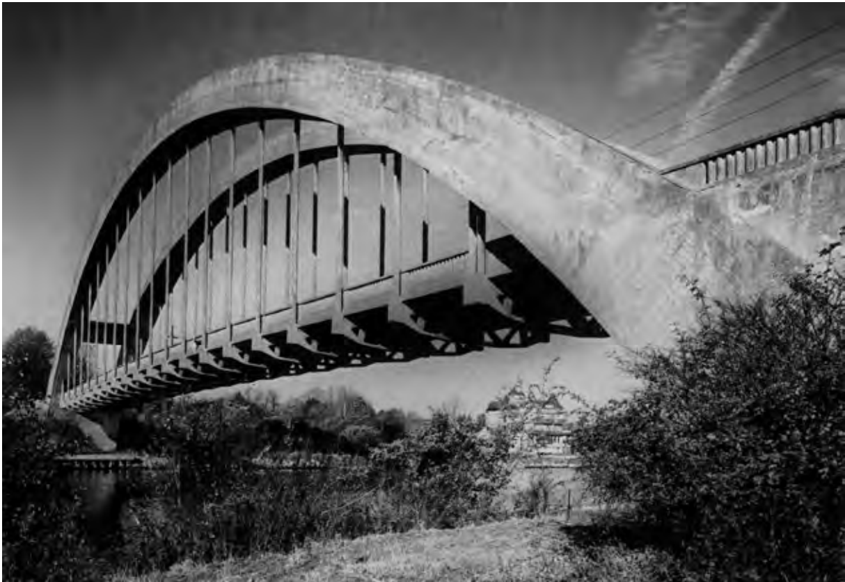
Figure 21 St. Pierre-de-Vauvray Bridge
