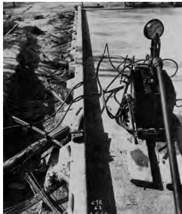
Figure 44 Luzancy Bridge, prestressing jack
