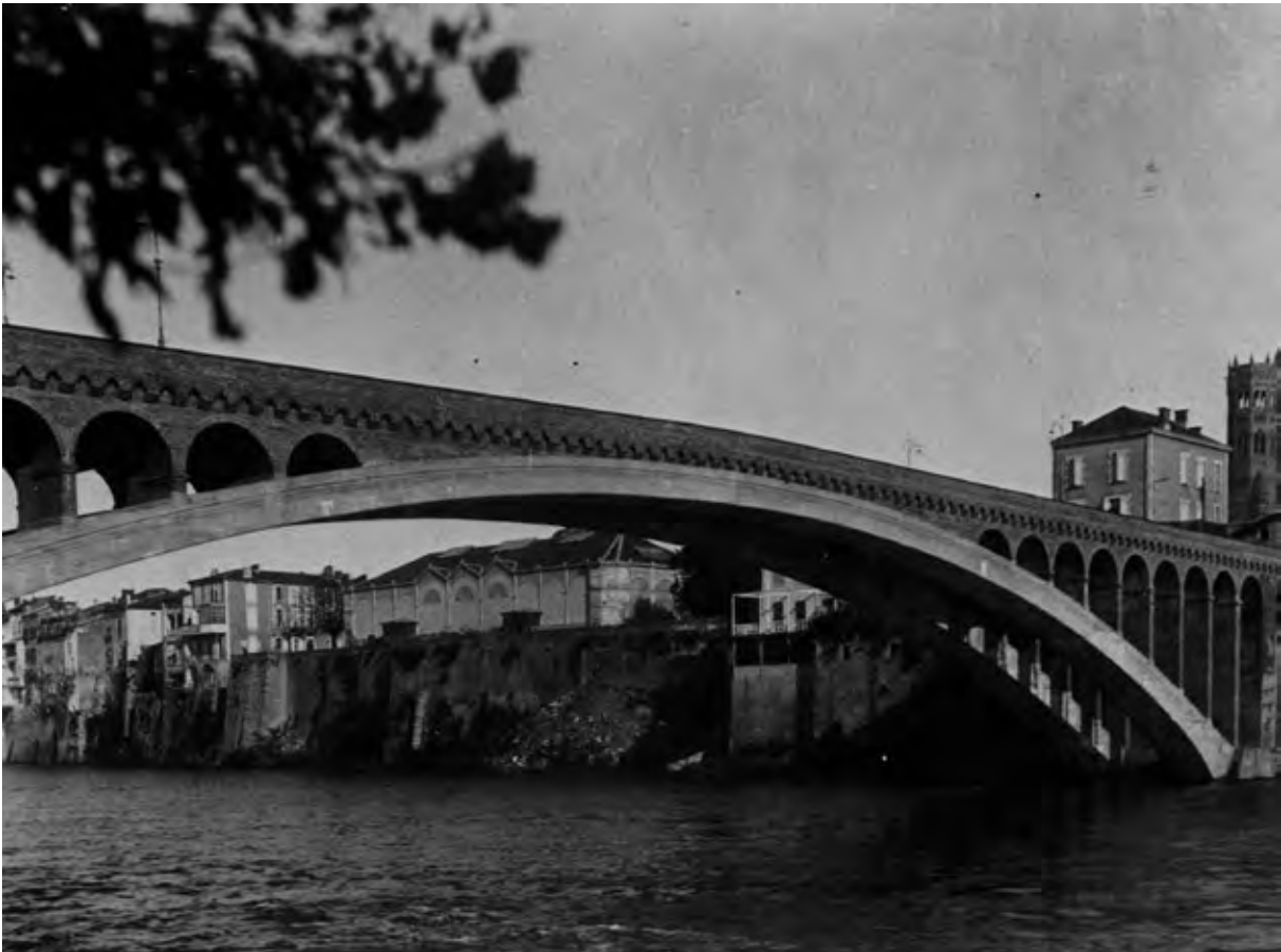
Figure 20 Villeneuve-sur-Lot Bridge finished
