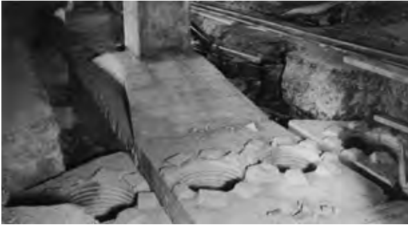
Figure 37 Detail of holes for the piles at the Maritime Station of Le Havre, solution for rehabilitation by Freyssinet in 1934
