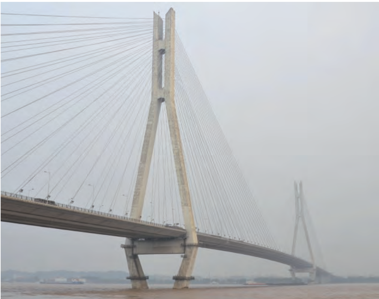
Fig. 3 Second Nanjing Bridge across Yangtze River
