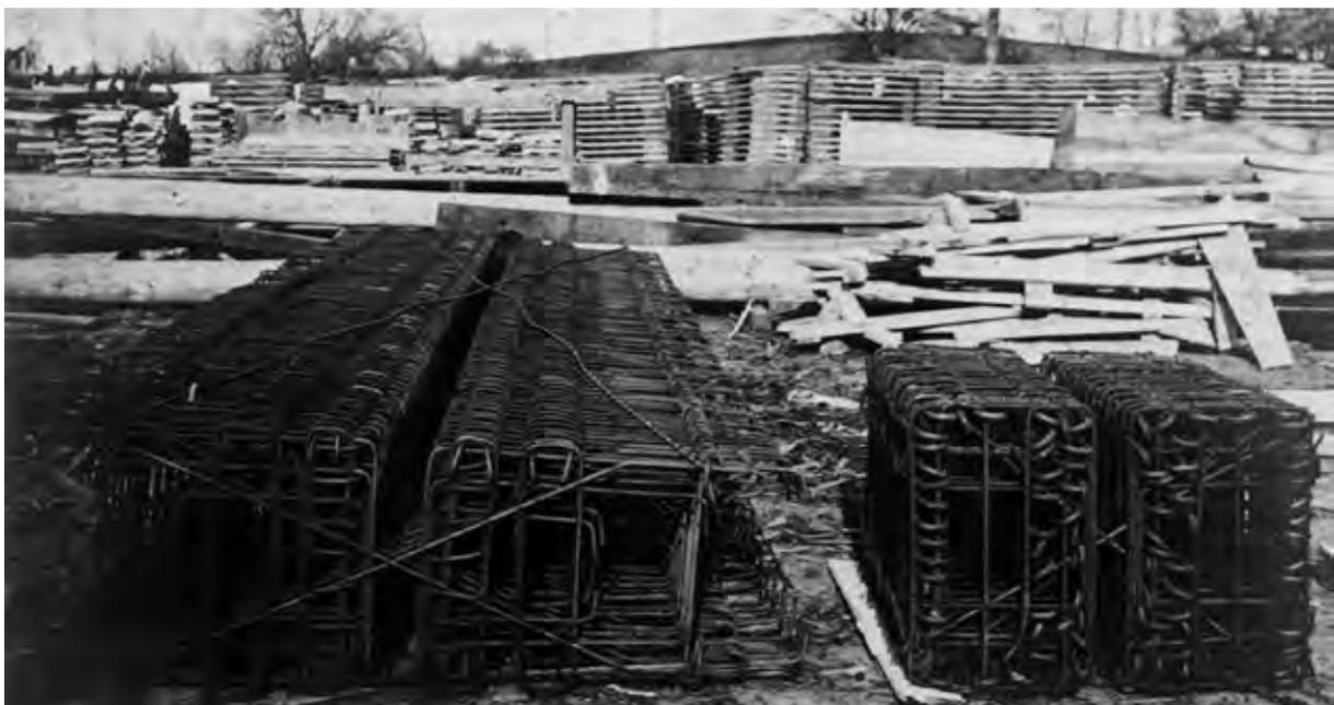
Figure 8 Boutiron Bridge, hinge reinforcement
