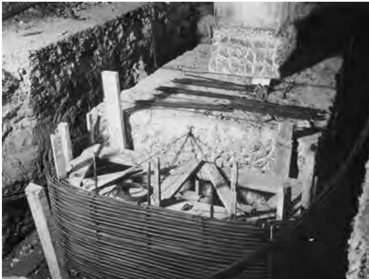
Figure 36 Anchor blocks at the Maritime Station of Le Havre, solution for rehabilitation by Freyssinet in 1934
