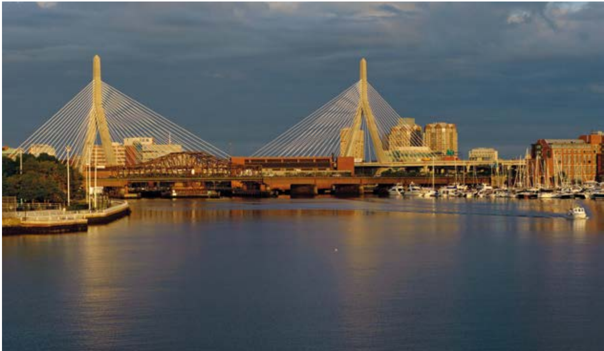
Bild 4 Leonard P. Zakim Bunker Hill Memorial Bridge in Boston Foto: von Eric Vance, USEPA Environmental-Protection-Agency – August 4, 2011 beautiful Boston vista, Gemeinfrei, https://commons.wikimedia.org/w/index.php?curid=51971978
