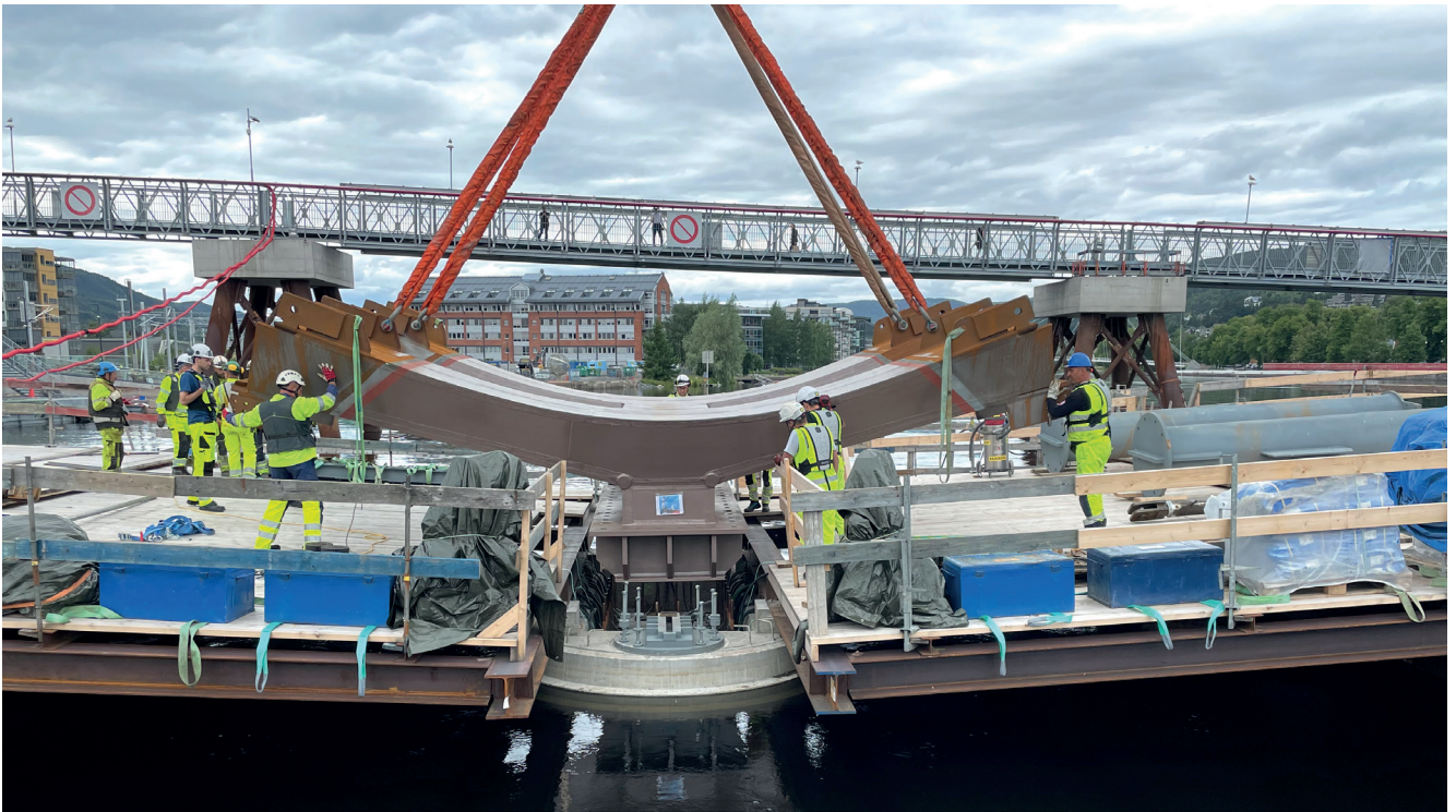
Figure 4: Erection of the steel fixed support on concrete pier at axis 7
