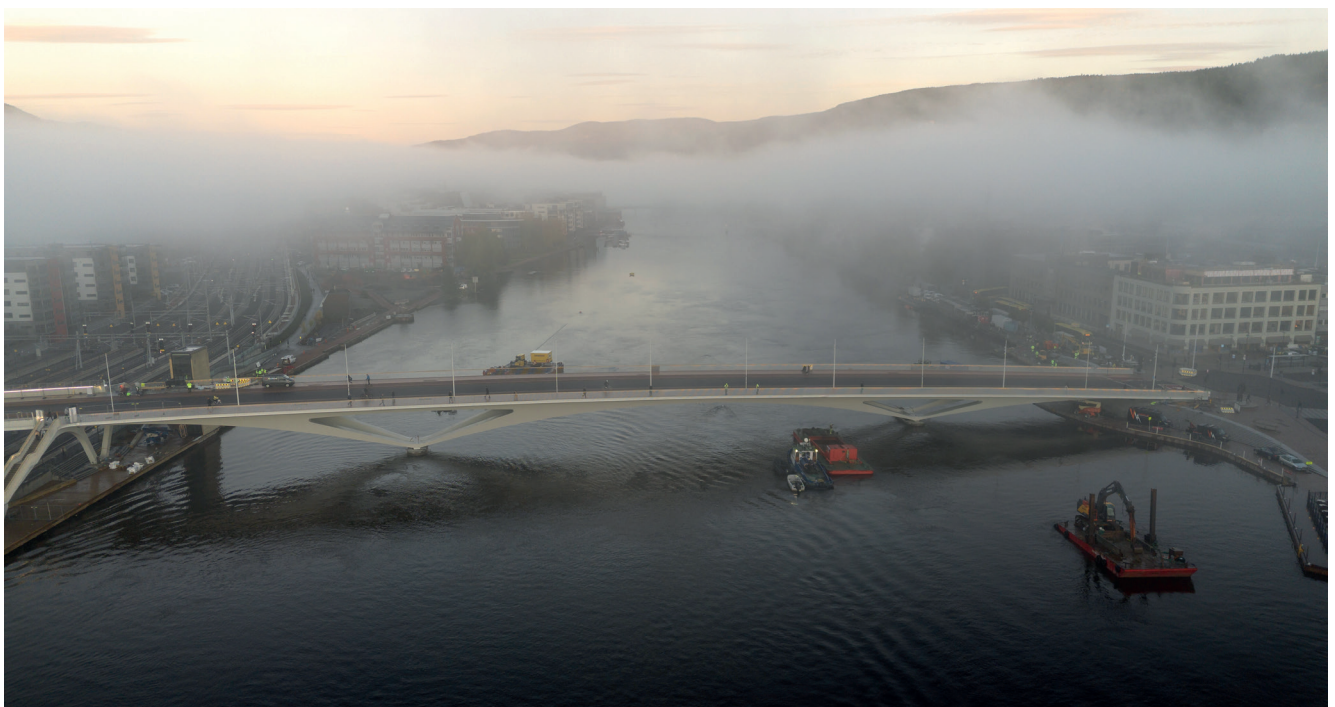
Figure 3: Overview of the bridge over Drammen River
