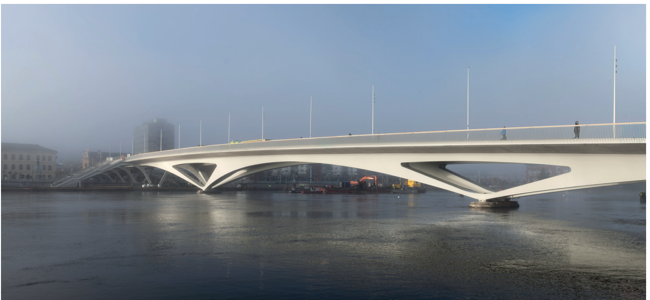
Figure 5: Lateral view of the finished bridge in service
