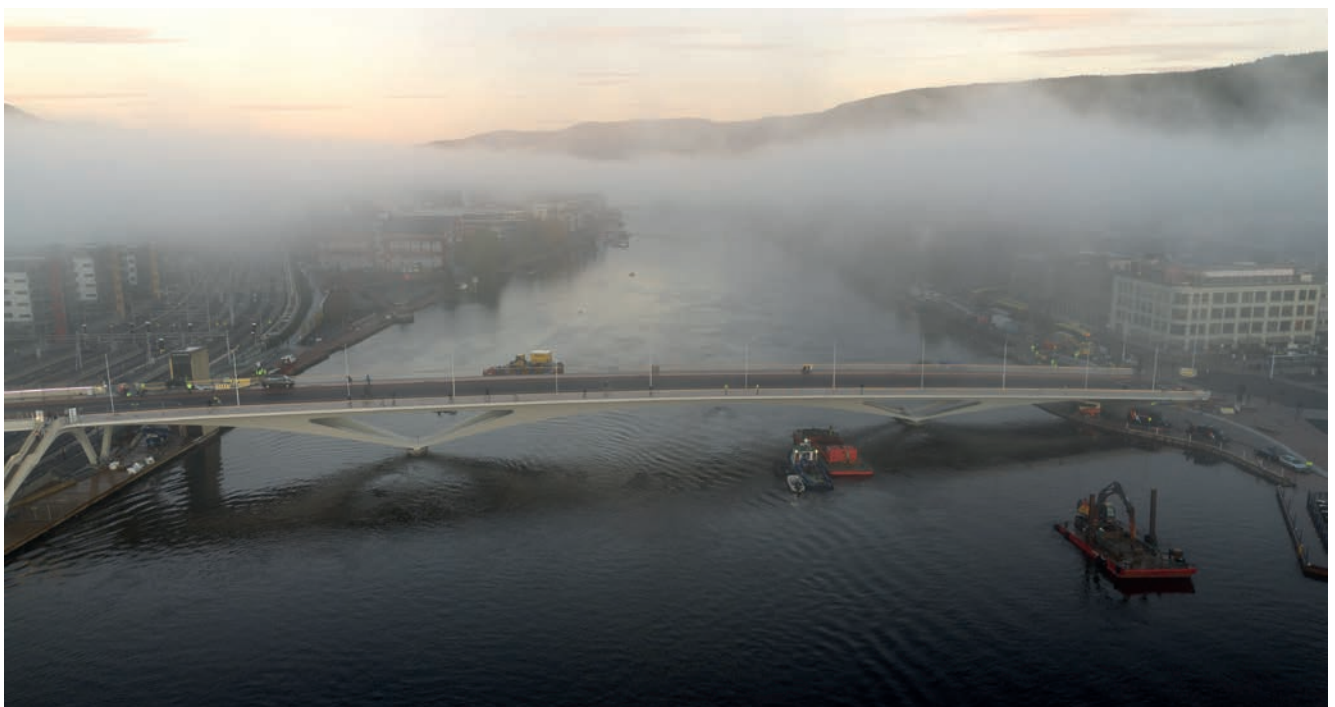
Figure 3: Overview of the bridge over Drammen River
