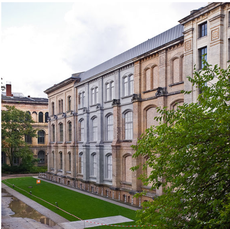
Fig. 10.12 Partly destroyed façade of eastern wing supplemented by concrete casts (with permission from Museum für Naturkunde—Leibniz Institute for Evolution and Biodiversity Science; photo: H.J. Götz)
