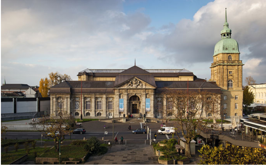
Fig. 20.1 Southern view of the museum building of the Hessische Landesmuseums Darmstadt in 2014 (with permission from HLMD; photo: Steffen Harms)
