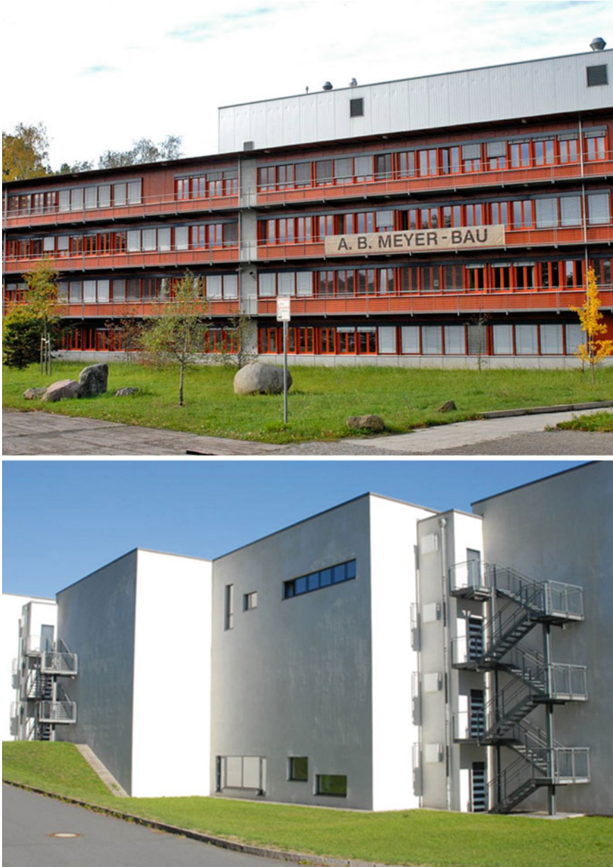
Fig. 28.30 A. B. Meyer Building, one of the new research and collection facilities of the Senckenberg Natural History Collections Dresden (with permission from: Senckenberg Naturhistorische Sammlungen Dresden (SNSD))
