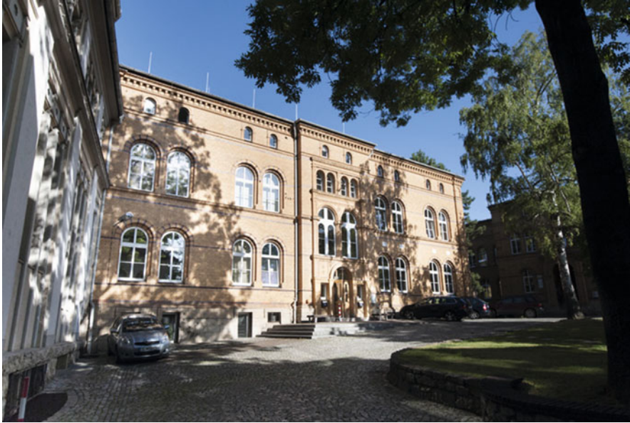
Fig. 37.1 The first zoology building in Wilhelminian style was opened in 1883. On the left, the second zoology building from 1912 which houses the zoological teaching collection until today (Photo: © with G. Brehm 2015)
