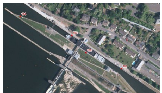
Figure 5: Locking chamber with 4 GPS-reference points which realized the reference system
