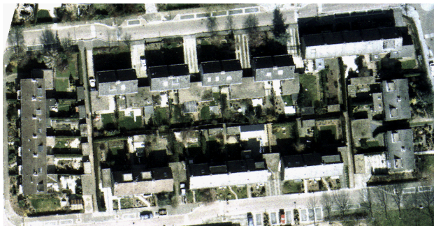
Figure 6: Aerial image of the region shown in Figure 5
