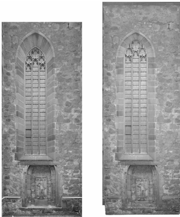
Figure 5. Projective transformation (left) and orthoprojection (right) of the same facade
