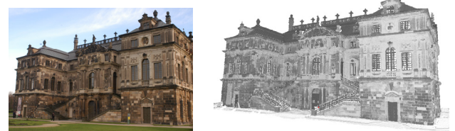
Figure 7. Image 112 (left) and point cloud (right) acquired from scan pos 4
