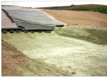
Surface sealing during construction
