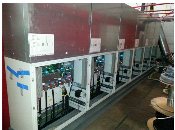
Fig. 6: (left) Assembly of the 3.2 MW prototype at the DyNaLab facility. (right) One “converter system” with 6 converter modules.
