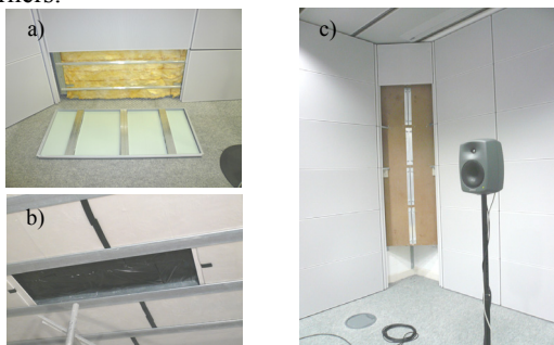
Figure 2: a) Mineral fiber treatment b) Plastic foil & min. fib. on ceiling c) Helmholtz resonator at the corner
