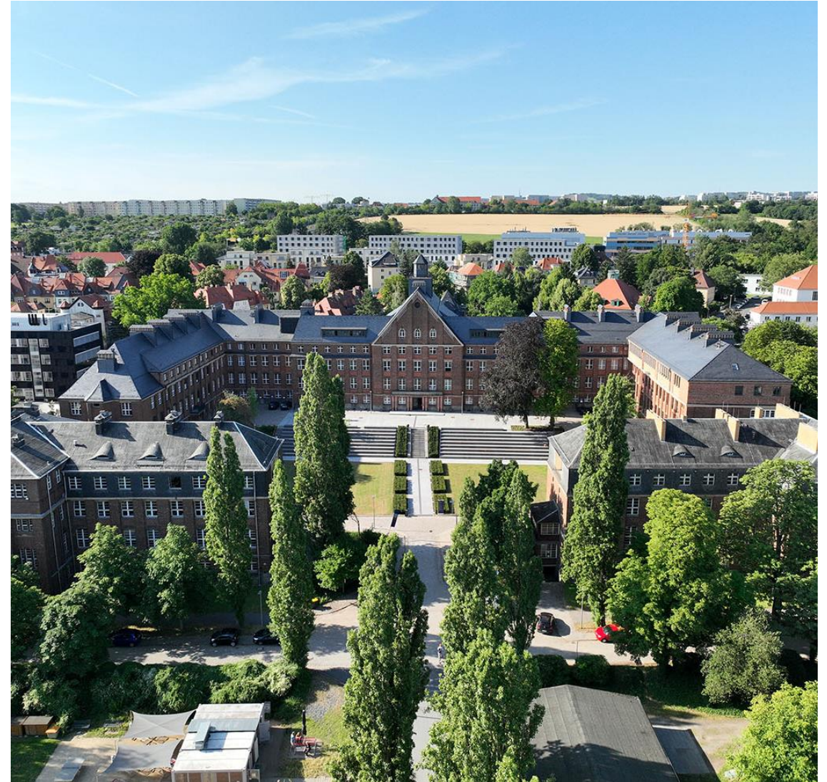
Service and support offers Fritz-Foerster-Bau
