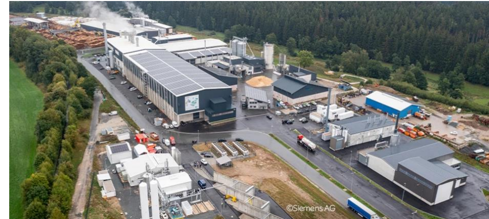
Energiepark Wunsiedel, Bavaria, Germany [6]
