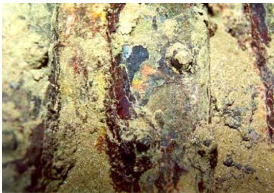
a) corrosion of a membrane wall under a SiC30 mass [6]
