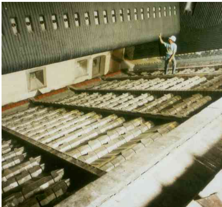
Fig. 1. MARTIN® reverse-acting grate for the combustion of difficult fuels [3].
