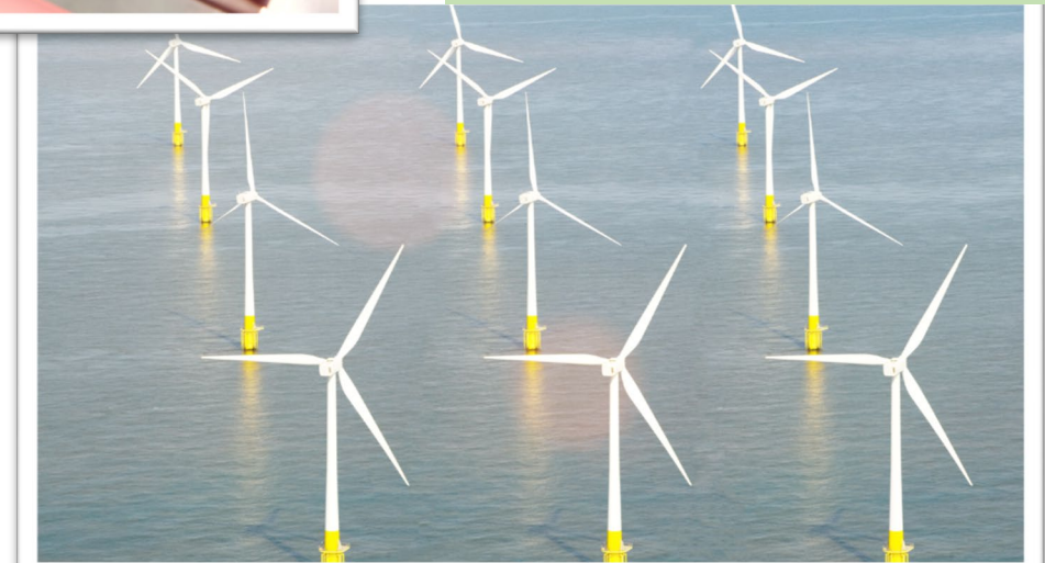
Industrial Power Control
